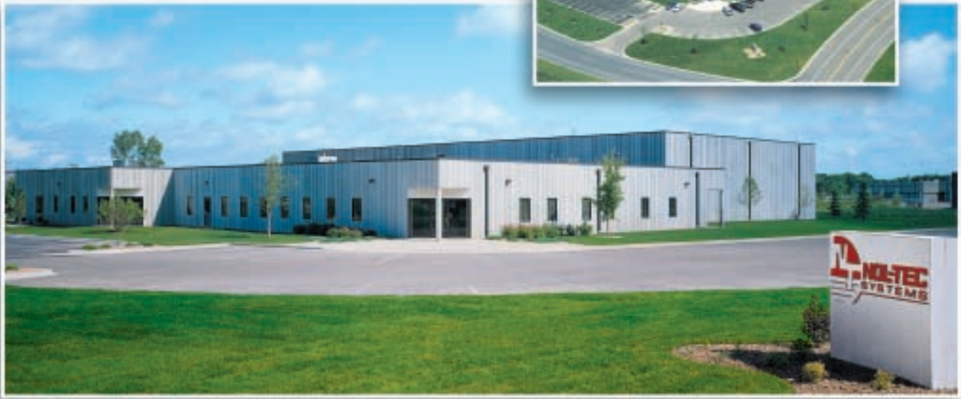
Corporate Headquarters, Lino Lakes (Minneapolis), Minnesota
